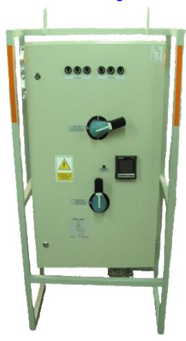
Through connection block type BPP2/1U/1 is a device designed for use in underground mining pits in non-explosive coal dust conditions and on the ground.
